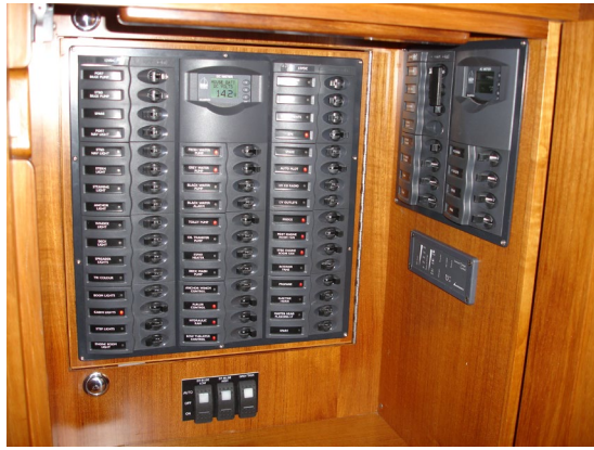
Hidden electrical panel
